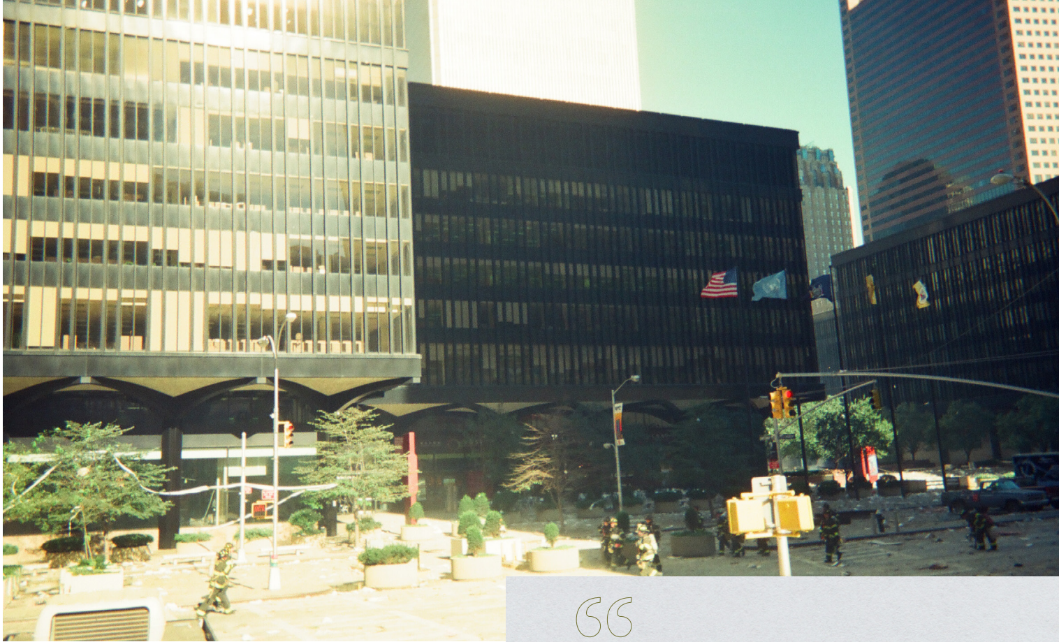
The 4 World Trade Center building on Church Street.
